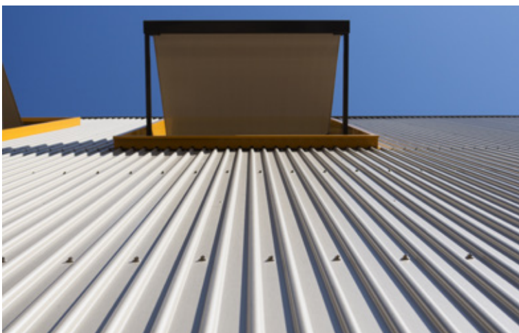
Each panel was formed in a complex pressing operation to create long, clean lines.
